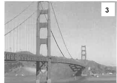
Golden Gate Bridge, San Francisco
